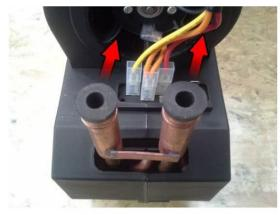
Drill necessary holes into the rear glove box cover and lead the hot water hoses and the heater harness through(red circles).
