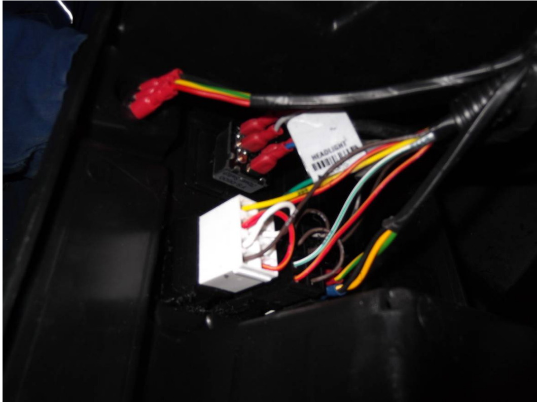
Inner view onto connected switches.
