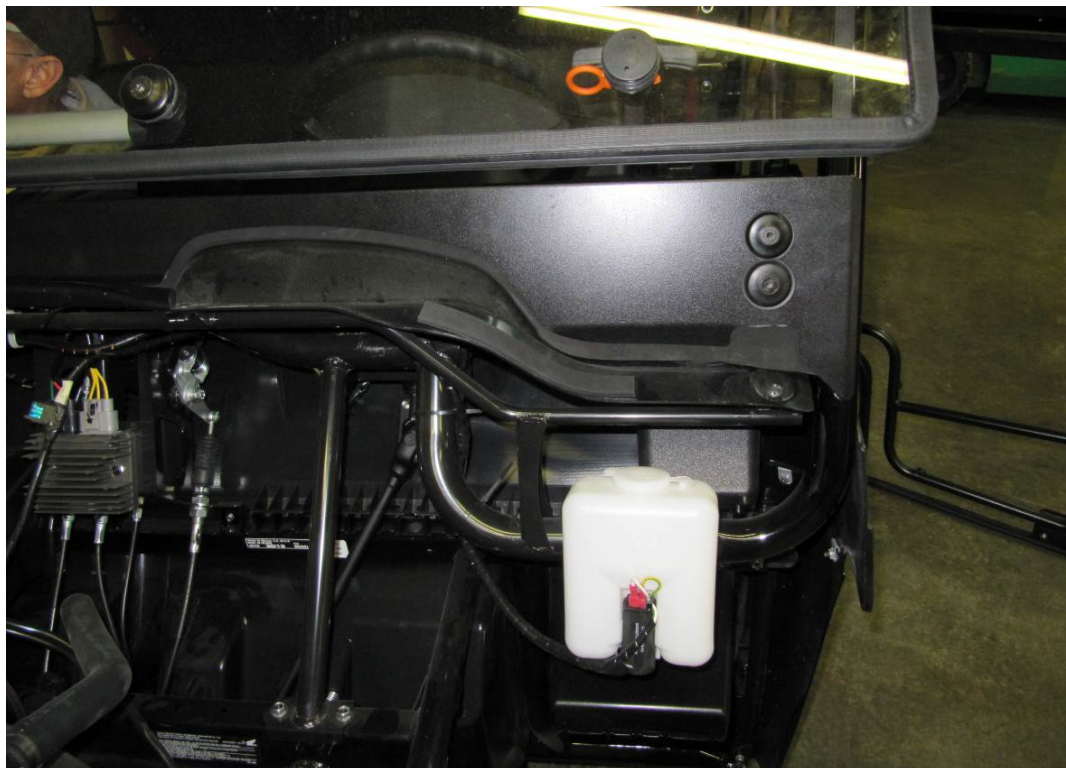
Lead the harness (red arrows) from washer tank to the main forklift switch electrification.
